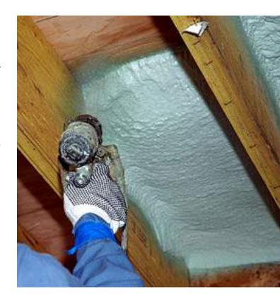
Spray foam insulation doesn't shift, settle or fall and lasts for decades beyond any fiberglass installed in your joists.
